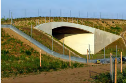
Figure 11: Greenbridge on the Austrian highway A6.
