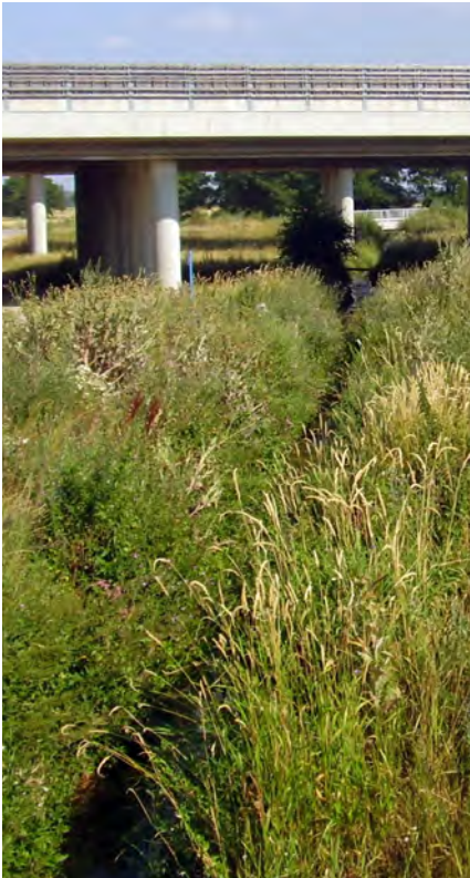
Figure 12: A bridge providing space to maintain the corridor functions of the underlying habitat.
